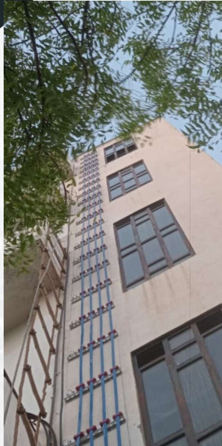
EARTHING STRIP WITH SLEEVE
